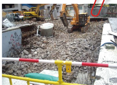
Demolition and foundation works
